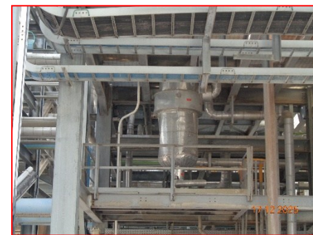
(8) Second Process Water Heater บริเวณ Vent Scrubber
